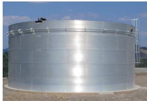
Fig. 3. A 24ft (7.3m) prefabricated metal tank. This design is a potentially lower cost alternative to molded plastic tanks. The metal cylinder serves as a frame to support a light tight bladder that stores the water. Though this tank is attached to a concrete pad, HAWC tanks will be buried about 1ft deep.
