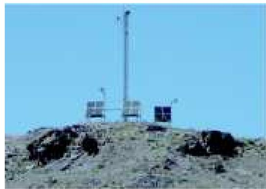
Fig. 2. One of the communication tower located at a hill called Smelter Knoll(SK). Three stands with four solar panels are seen.
